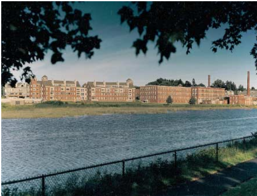
The same view, after renovations and the new construction were complete.
